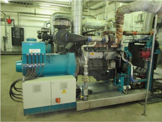
Fig. 2. Demonstration of a co-generation unit in the BS 1 biogas station
